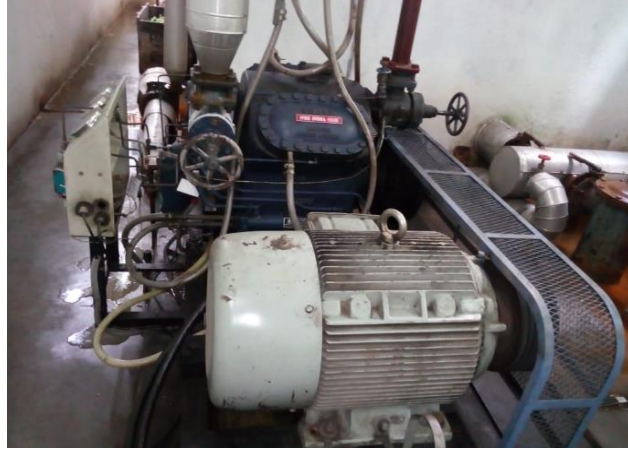
Figure 5: Chiller Compressor
